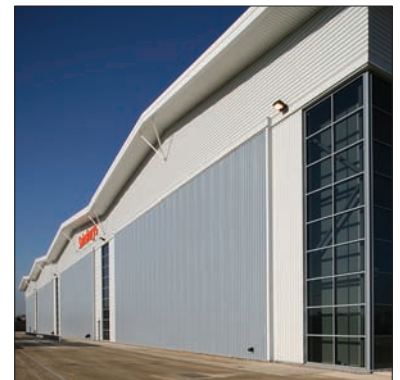
SolarWall system by Conserval Engineering at Sainsbury Distribution Centre, Pineham. Source: SolarWall
