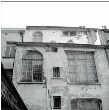
Façades prior to refurbishment Renewable Energy House, Brussels. Source: EREC
