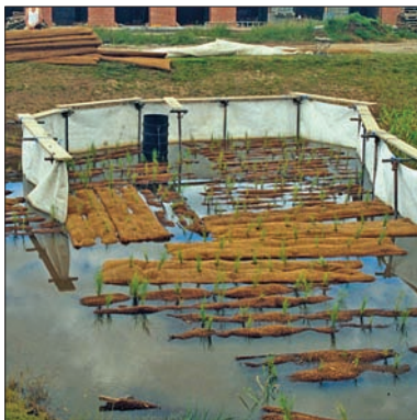
Constructed wetlands, Hockerton Housing Project, Nottinghamshire. Source: Hockerton Housing Project Trading Limited
