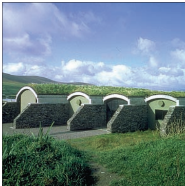
Grass roof on the Skellig Intepretive Centre, Ireland. Architects: Peter and Mary Doyle
