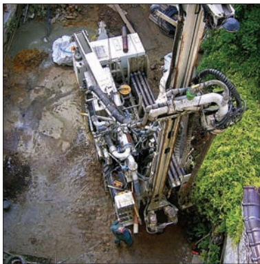
Drilling a Borehole. Source: Passivhaus Institute Darmstadt
