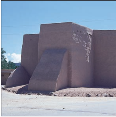
Rammed earth construction, Mexico
