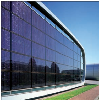
Integrated photovoltaic façade in Tobias Grau GmbH Head office, Rellingen. Architect: BRT Architects. Source: Schueco International KG
