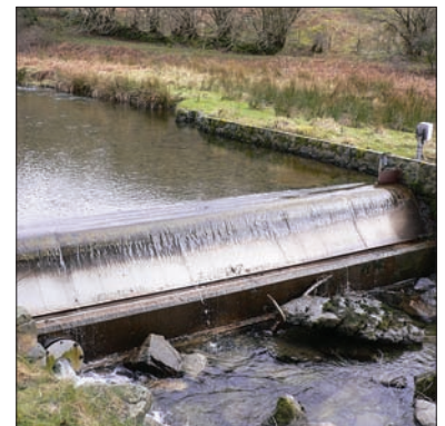
Small scale hydro plant. Source: Dulas Ltd
