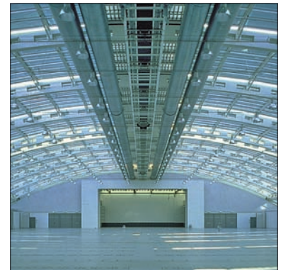
Light directing glazing at the Design Centre, Linz. Architect: Herzog and Partner Architects
