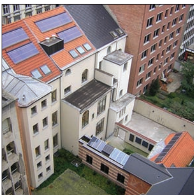
Refurbished Renewable Energy House, Brussels. Source: EREC
