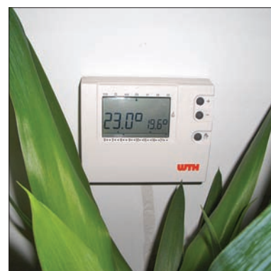
Heat recovery ventilation control unit. Source: Passiefhuis Platform VZW (PHP)
