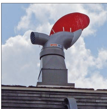
Passive ventilators with heat recovery, Bedzed, London. Source: Andrea Rota
