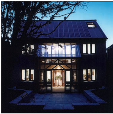
Photovoltaic roof, Roaf House, Oxford. Architect: S. Roaf
