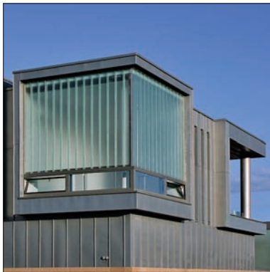
Zinc cladding, Model Arts and Niland Gallery, Sligo. Architect: McCullough Mulvin Architects
