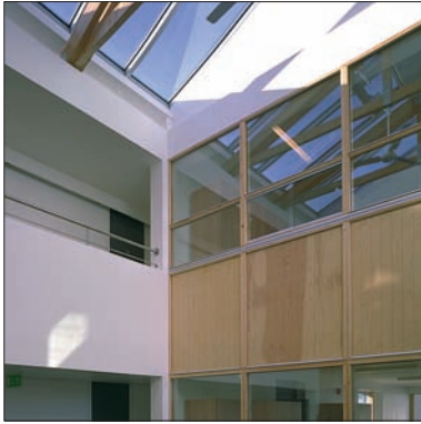
Softwood timber panelling, the Irish Energy Centre, Dublin. Architects: UCD Energy Research Group, University College Dublin
