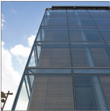
Double skin façade, Riverside, Dublin. Architect and source: STW Architects
