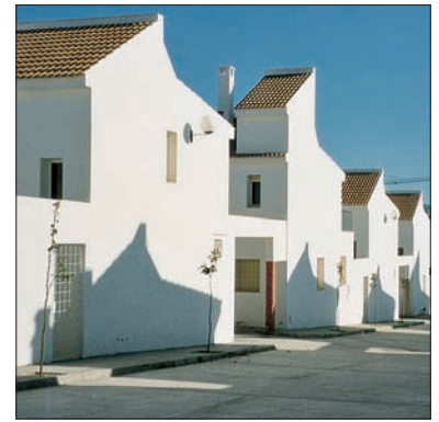
Pale surfaces reflect solar radiation. Architect: Sottomayor, Dominguez and Lopez de Asian
