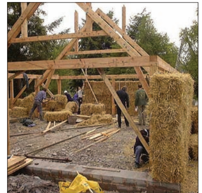
Straw bale construction at the Centre for Alternative Technologies (CAT), Wales. Source: CAT
