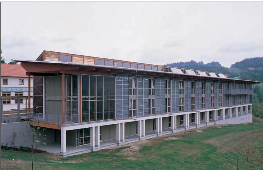
Hostel at Windberg with transparent insulated façade. Architect: Herzog and Partner Architects
