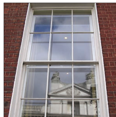
Secondary glazing. Source: Zsuzsa Szalay
